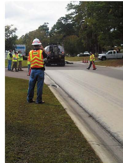
South Carolina DOT staff observes placement of Reclamite rejuvenator in Charleston County
